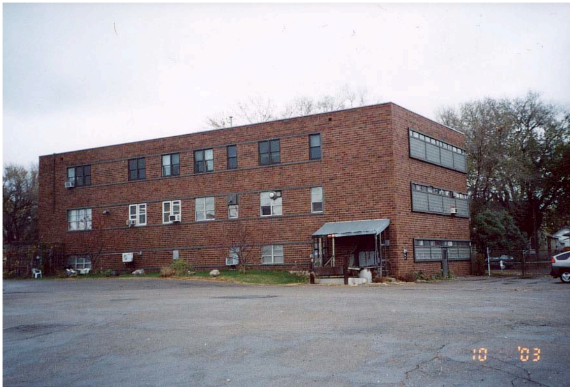
Back of Building 14
