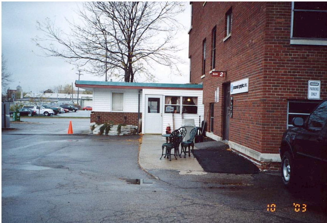
Guardhouse attached to Building 2
