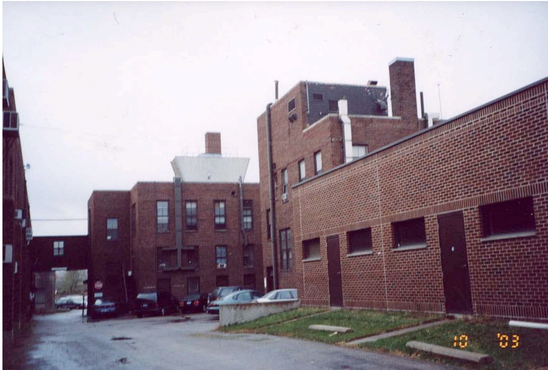
Front of Buildings 7, 8
