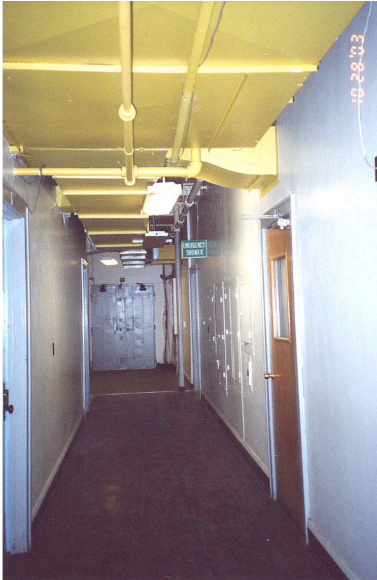
Hallway between buildings 10 and 7
