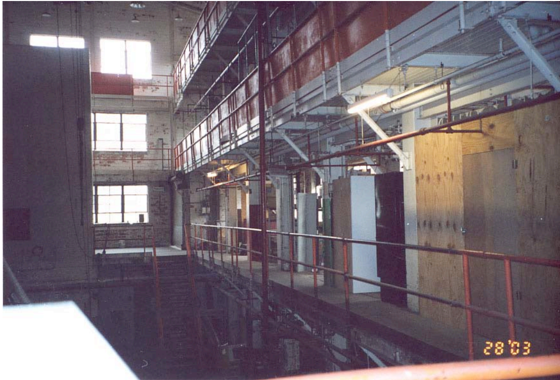
Interior of Building 10
